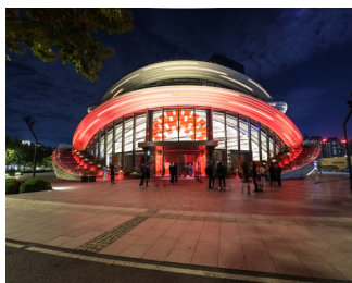
02 West Bund Central | The Orbit West Bund Shanghai art building ©Davide Colombino
