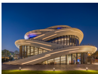
07 West Bund Central | The Orbit West Bund Shanghai art building
