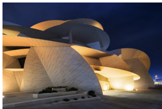
25 Lighting design for National Museum of Qatar Hervé Descottes ©Iwan Baan_L'Observatoire International
